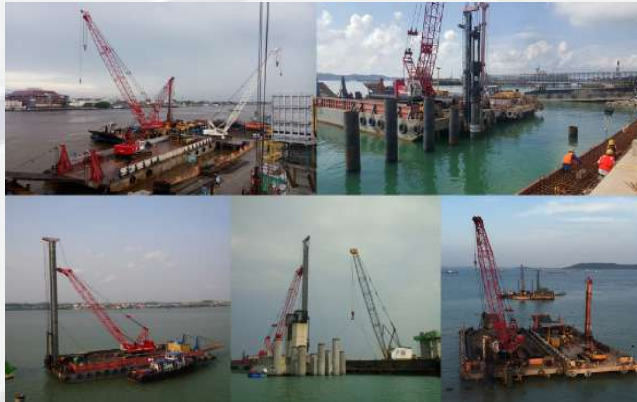
Foundation & Retaining Wall
