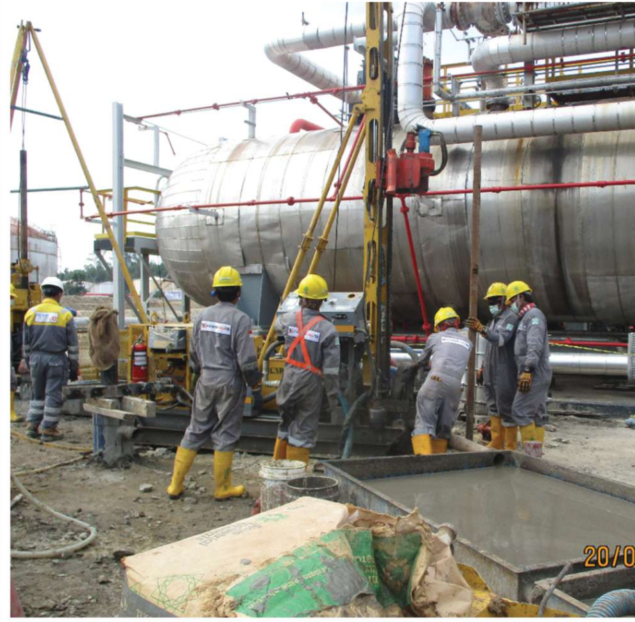
PT RDMP Balikpapan JO Micropile work on the Pertamina Refinery Development Master Plan (RDMP) Project in Balikpapan.
